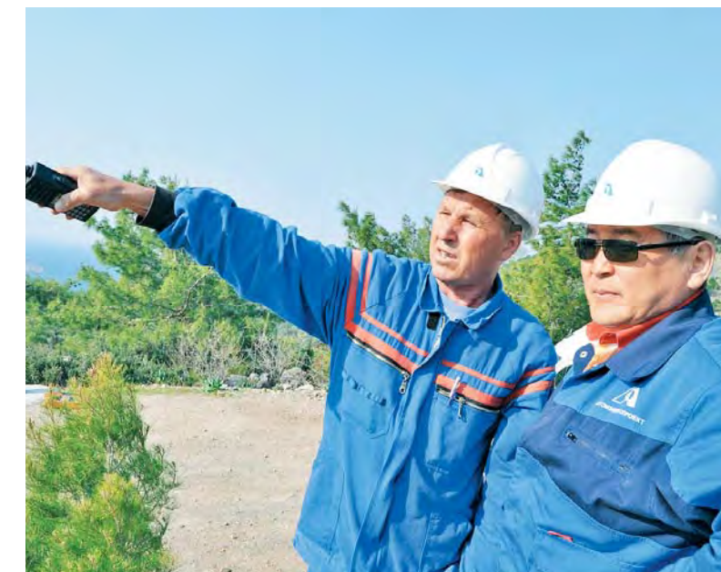
The employees of AEP at the Akkuyu NPP construction site during the engineering survey. Photo: Akkuyu Nükleer, 2012
